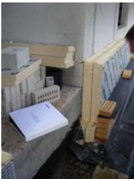
Insulation of walls.
