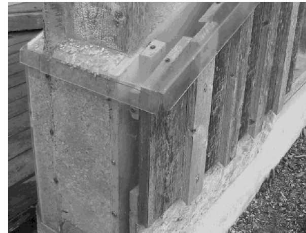
Figure 8: Out wall construction: cladding
