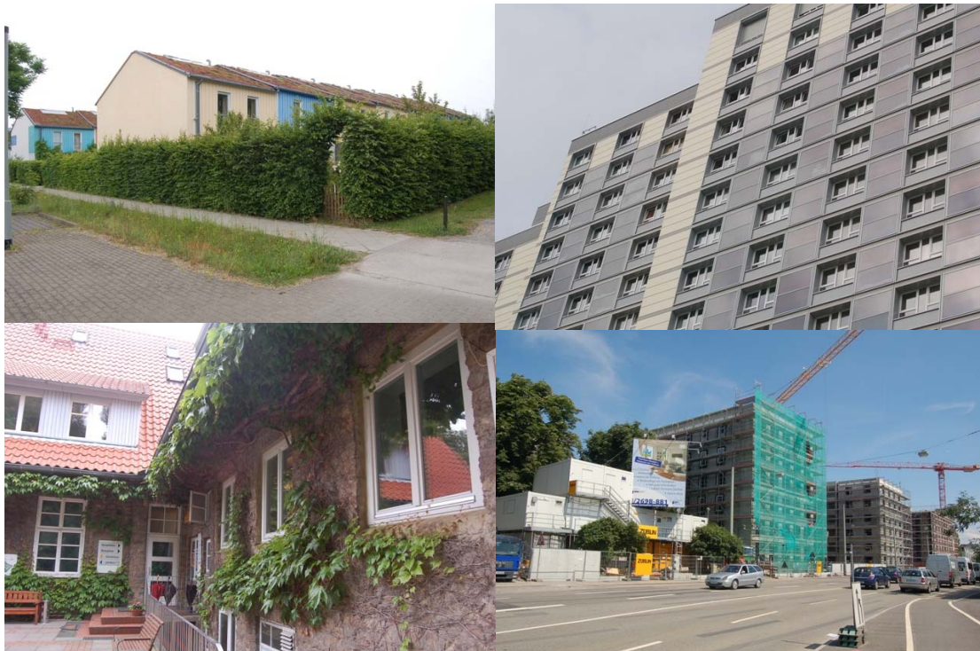
Picture 2.1: Different building types but reaching the same standard – passive house standard or low energy standard
