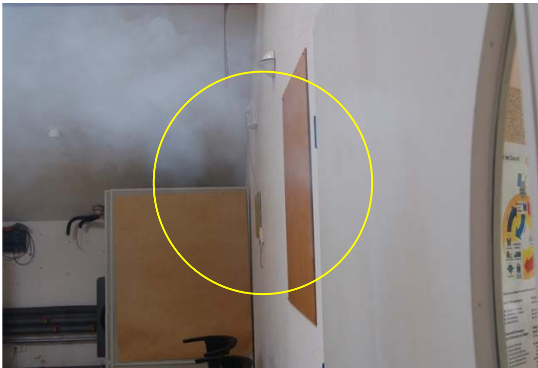
Picture 4.6 (e.u.z, Springe, Germany 2009): detail at the picture is indicating by smoke where is the flow of the air to the room.
