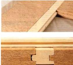
Tongue and groove joint for a floor construction
