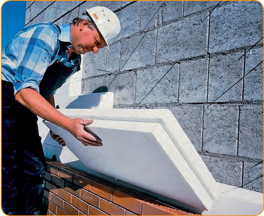
Fig. 2. Insulation of outer walls of a building Image: © Nikecell
