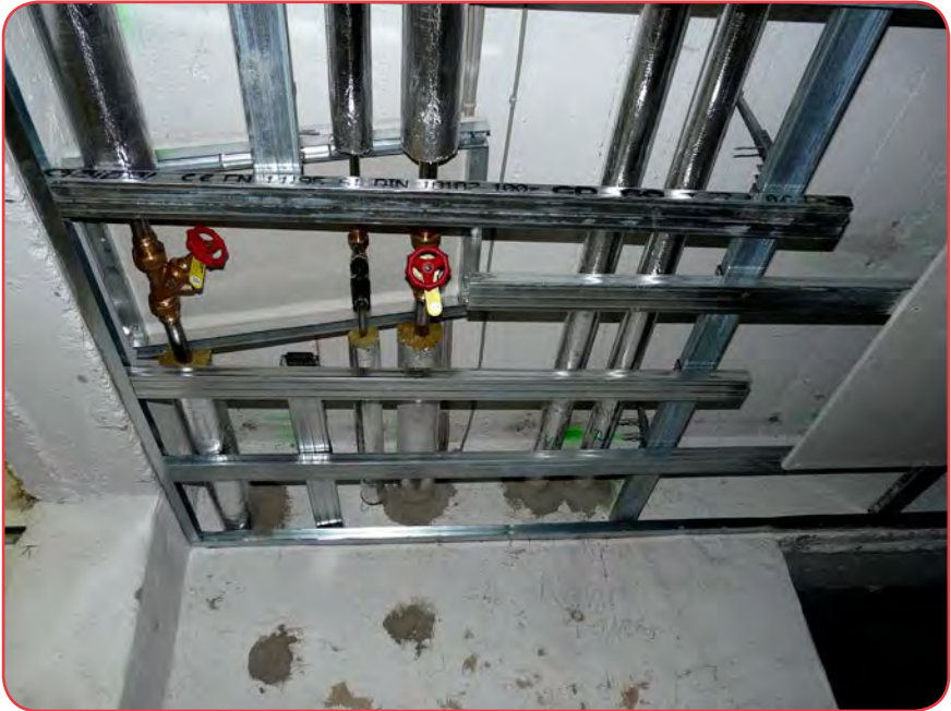
Fig. 7. Preparation for insulating the cellar ceiling Image: © Jörg Faltin
