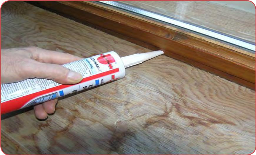
**Fig. 3.** Application of sealant on a window frame.
