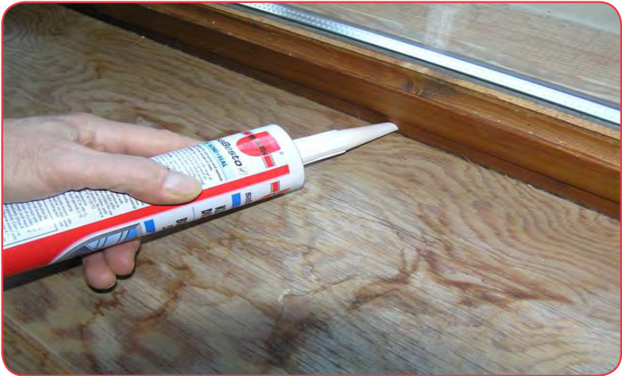
Fig. 3. Application of sealant on a window frame.
