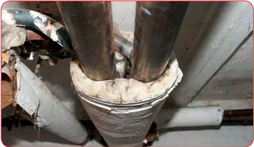
Fig. 1. Insulating your heat pipes ensures that the heat reaches your rooms rather than to get lost on the way | Image: © Philipp Engewald.
