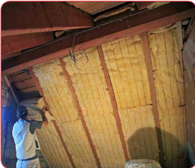
**Fig. 6.** Adding of rafter insulation to decrease the heat loss through the roof.
