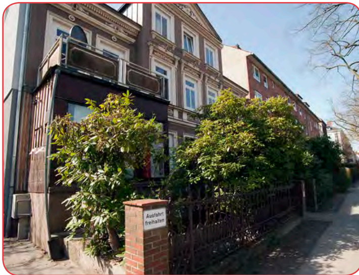
Fig. 8. Bushes and trees can be an effective heat protection. Image: © Philipp Engewald
