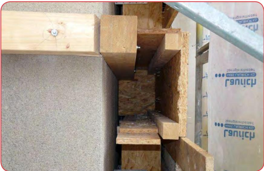
**Fig. 5.** Prepared wood casing on an outside wall to be later filled with insulation material | Image: © Jörg Faltn
