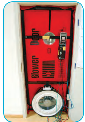
Fig. 4. Equipment to perform a blower-door test | Image: W. Walter
