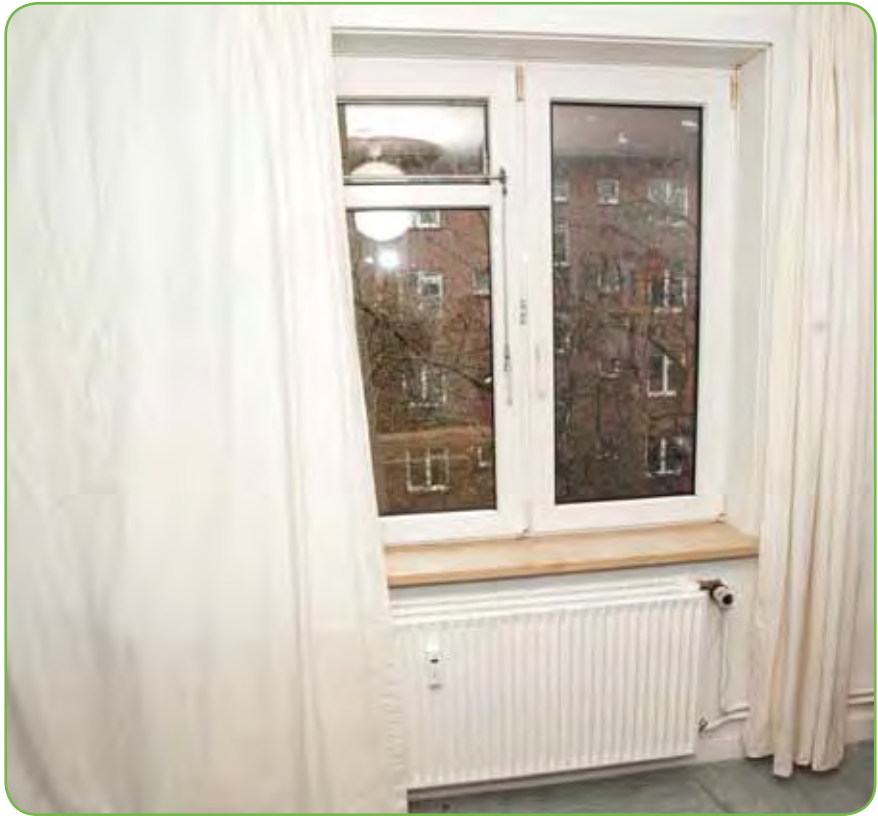
Fig. 1. Don't do it like shown here! Keep the radiators free from any furniture or curtains. | Image: © Philipp Engewald
